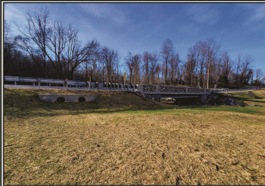
Post Construction - Bridge No. F09-25 and Additional Pipes for Overflow
