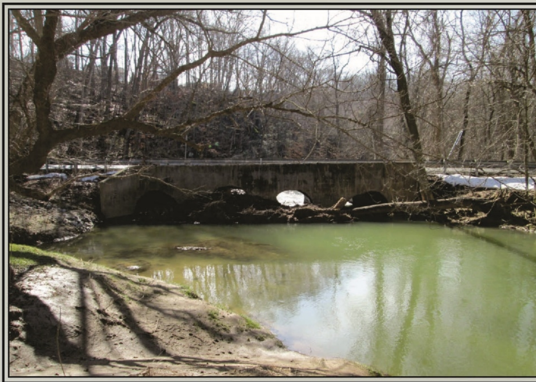
Pre Construction - Structure No. F09-21 Upstream End Blocked with Debris
