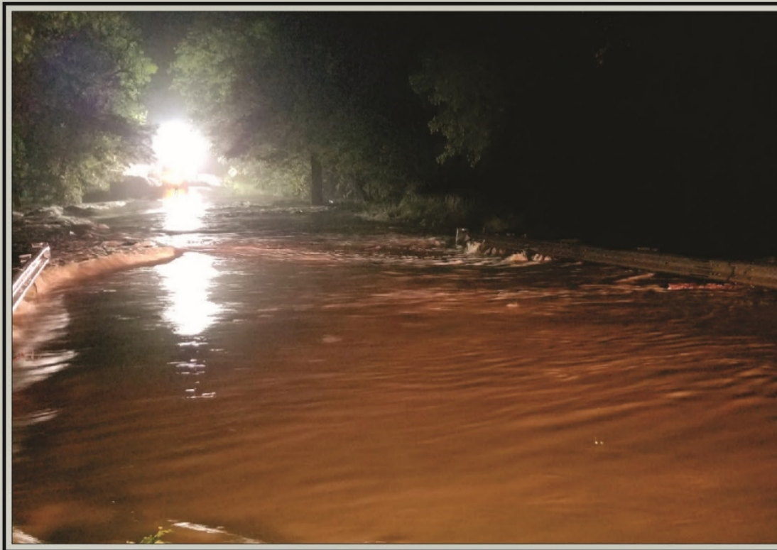
Pre Construction - Roadway Overtopped by Storm Event at Structure No. F09-21 and Smaller Structure
