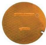
Full surface oxidation
