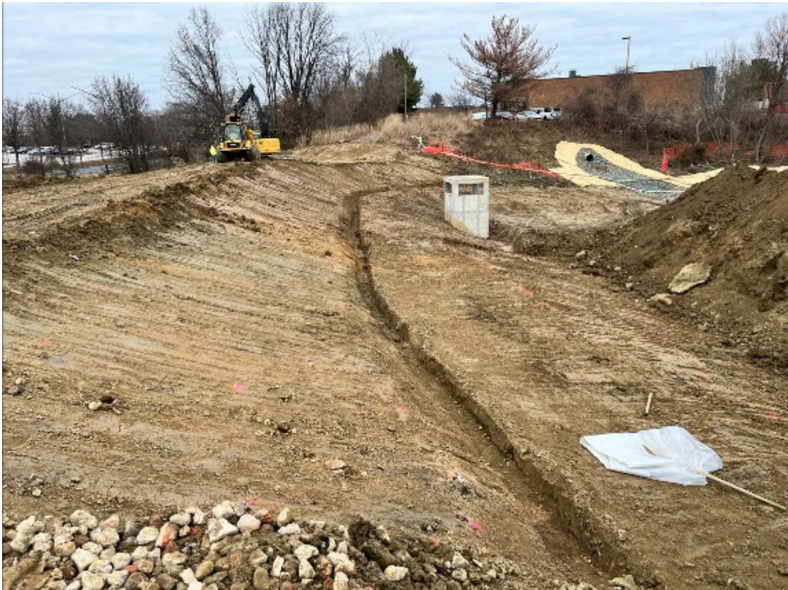
Anchor Trench Excavated During Fine Grading
