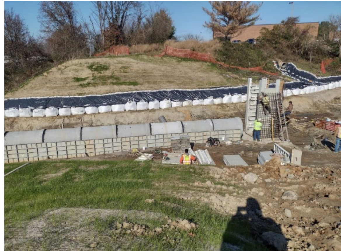
Segments of Reinforced Concrete Pipe and Formwork for Concrete Cradle
