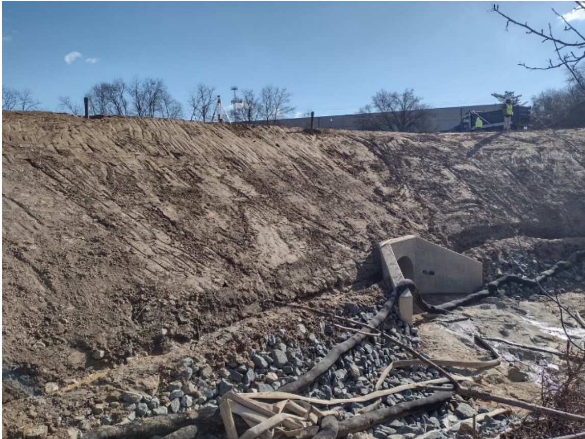
Fine Grading Before Subgrade Inspection
