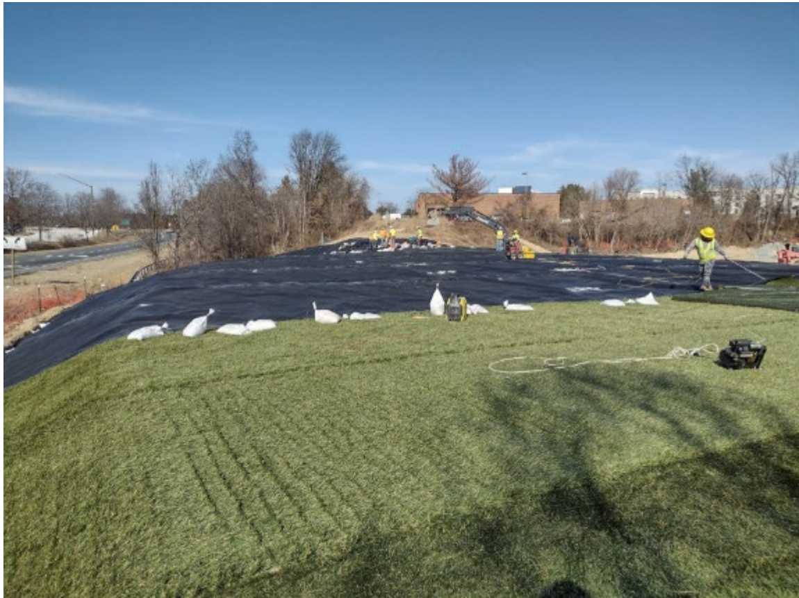
Pulled Out and Heat Bonded by Hand
