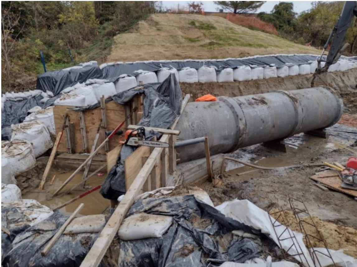
Segments of Reinforced Concrete Pipe and Formwork for Concrete Cradle
