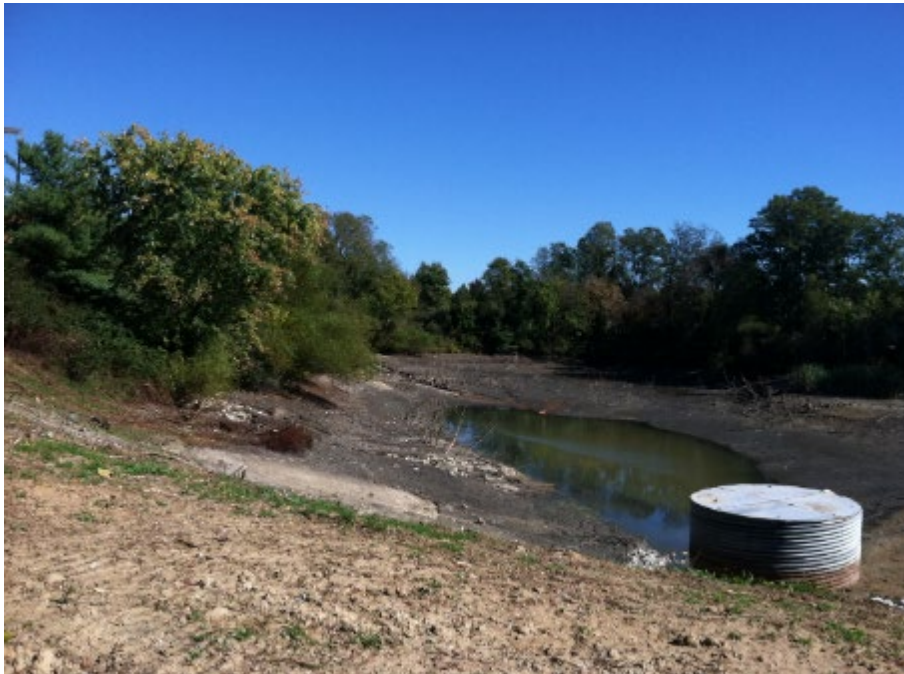
Site Prior to Retrofit
