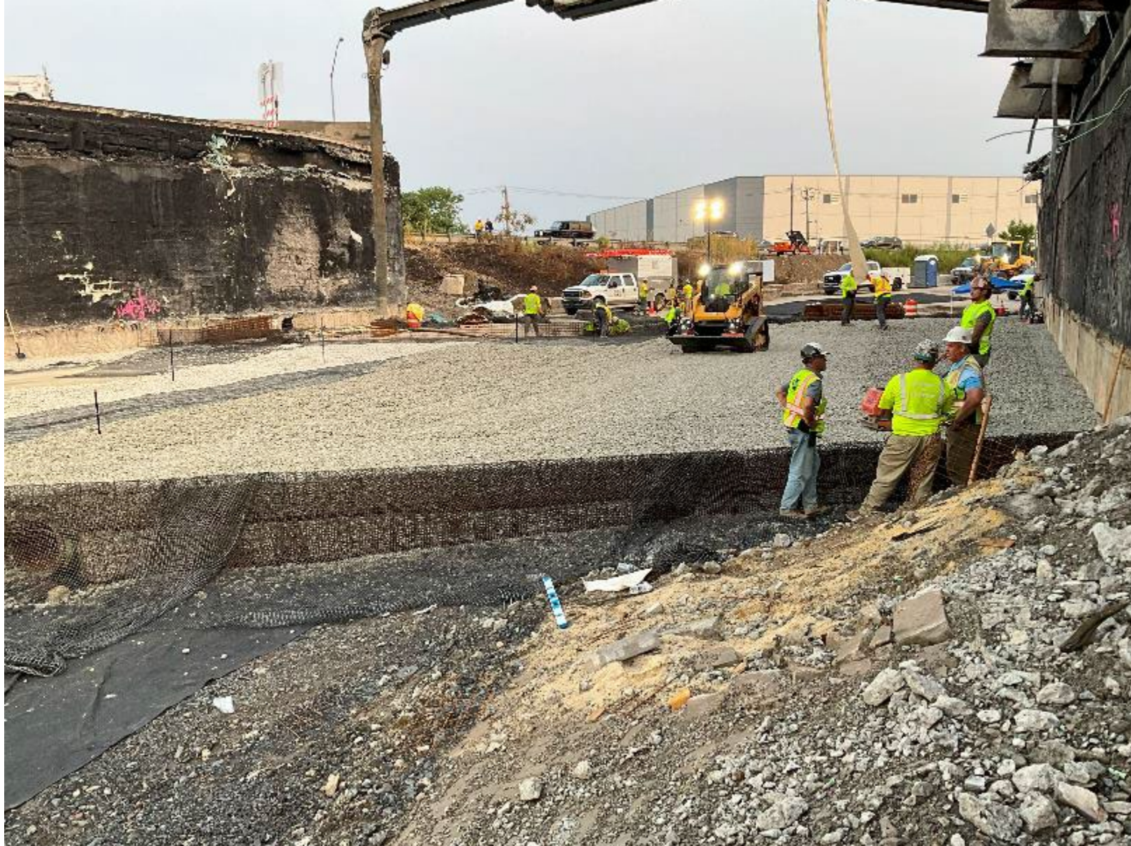
Compaction Skid Steer
