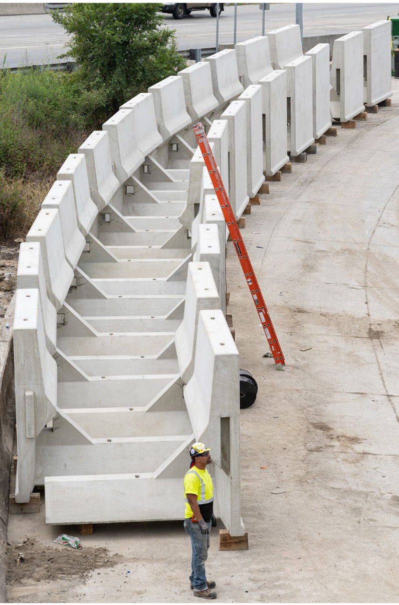
Precast Barrier Staging/ Placement
