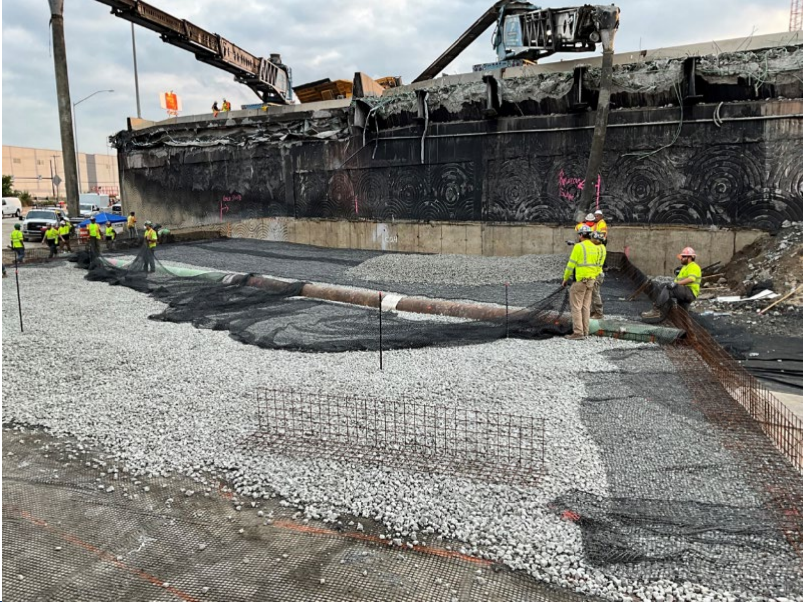
First Lift - MSE Wall Construction
