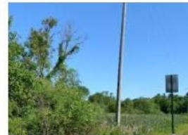
MW Quadrant with Electrical 20' West
