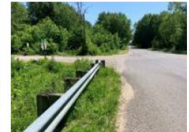
Intersection South of Bridge
