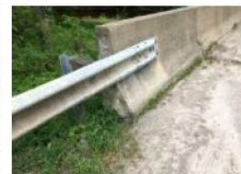
NE Corner of Deck
