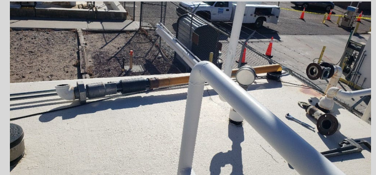
Inspection and functionality test of overfill prevention valves
