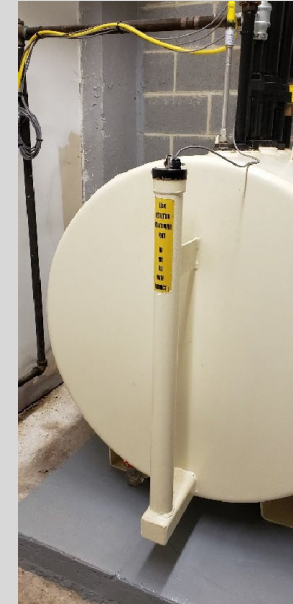
Interstitial Sensor (electronic)
