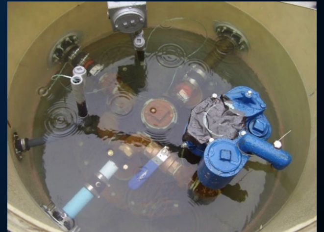
Submersible Turbine Pump Containment Sump
