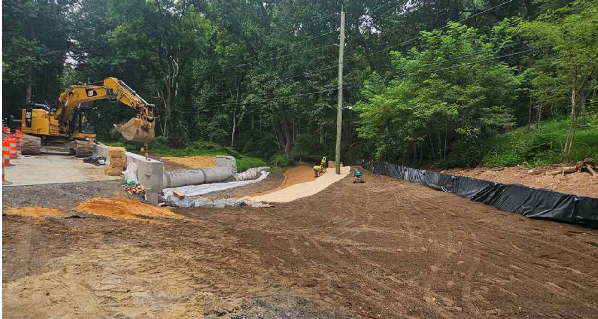
Bypass Road and Culvert Removal / Stream Grading and Stabilization
