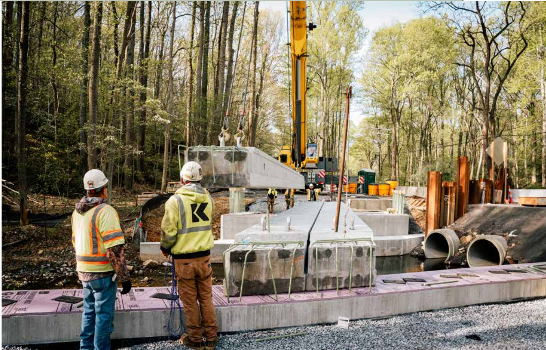
Prestressed Slab Erection
