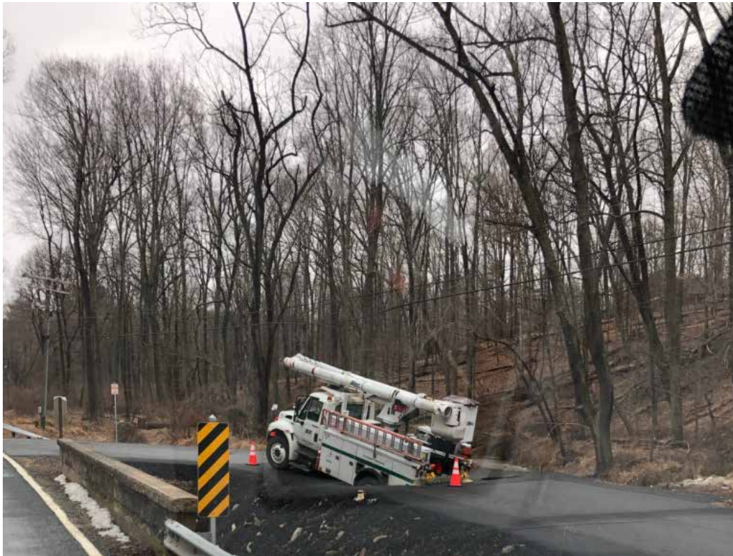
January 2021 – Washout and Pavement Failure
