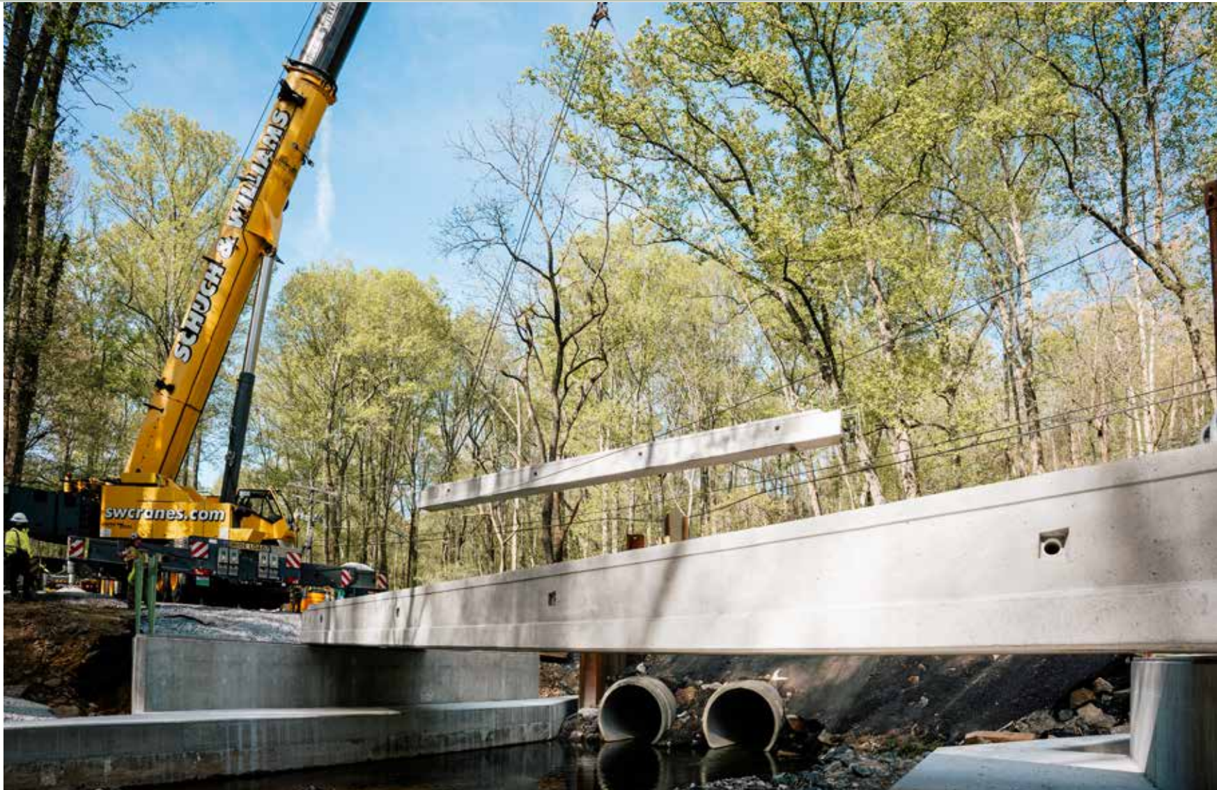
Prestressed Slab Erection
