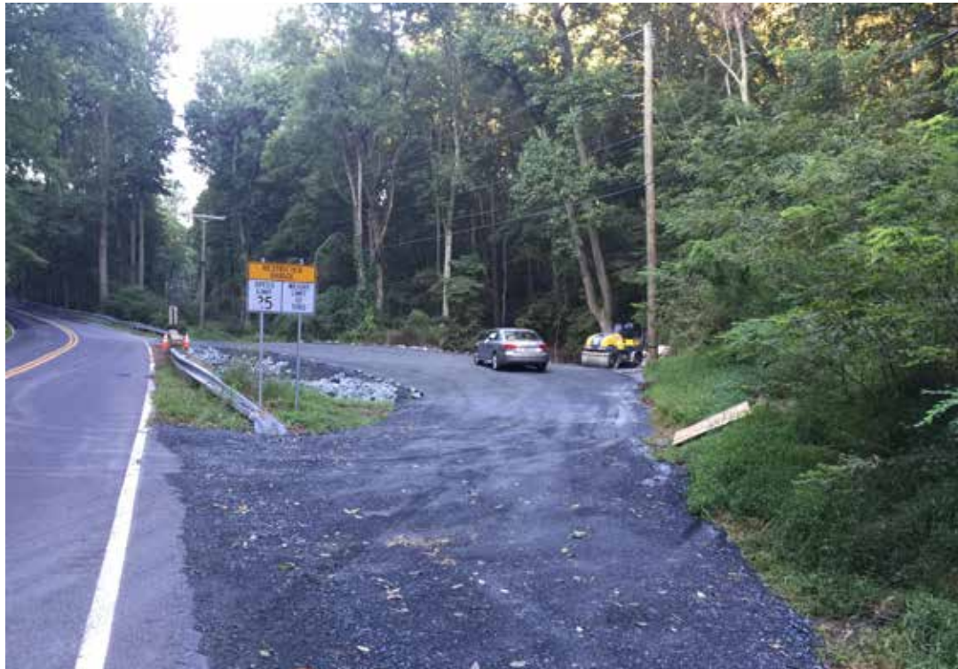
August 2016 – Emergency Repair
