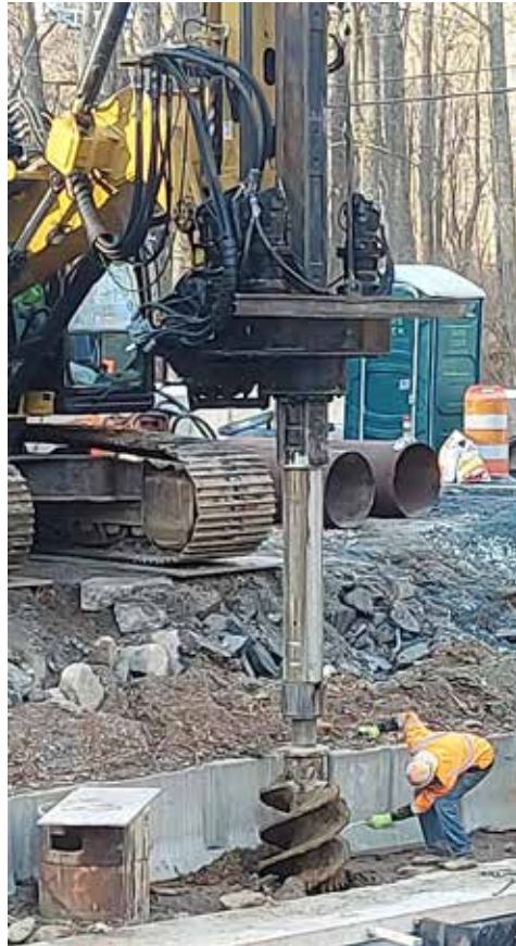
Drilled Shaft Foundations with Rock Sockets
