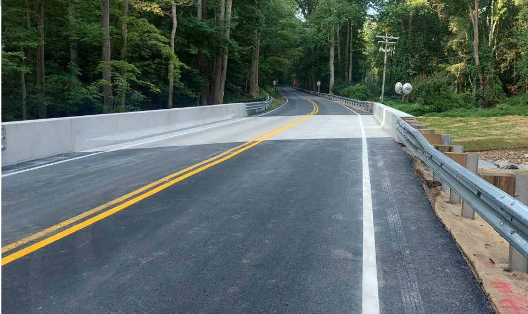
Final Paving and Line Striping
