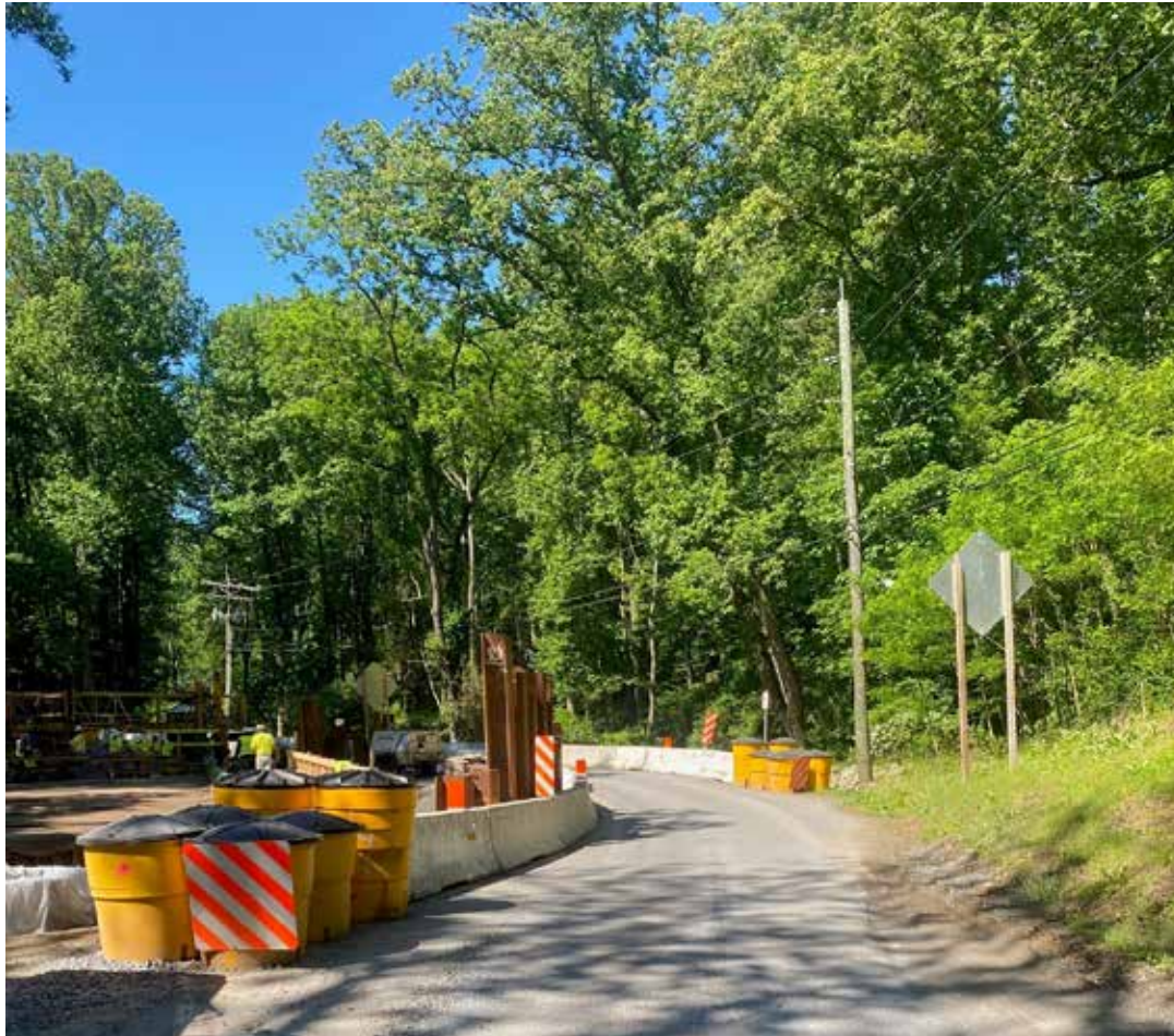
Bypass Road for Maintenance of Traffic / Temporary Support of Excavation
