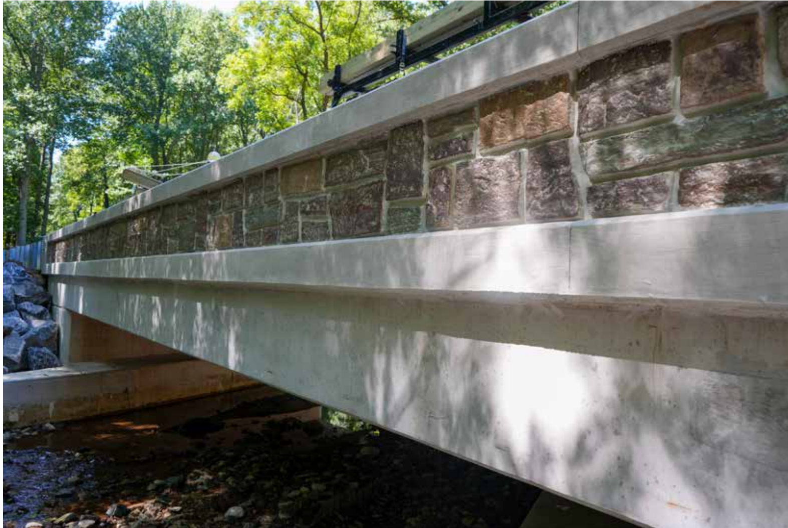
Simulated Stone Formliner
