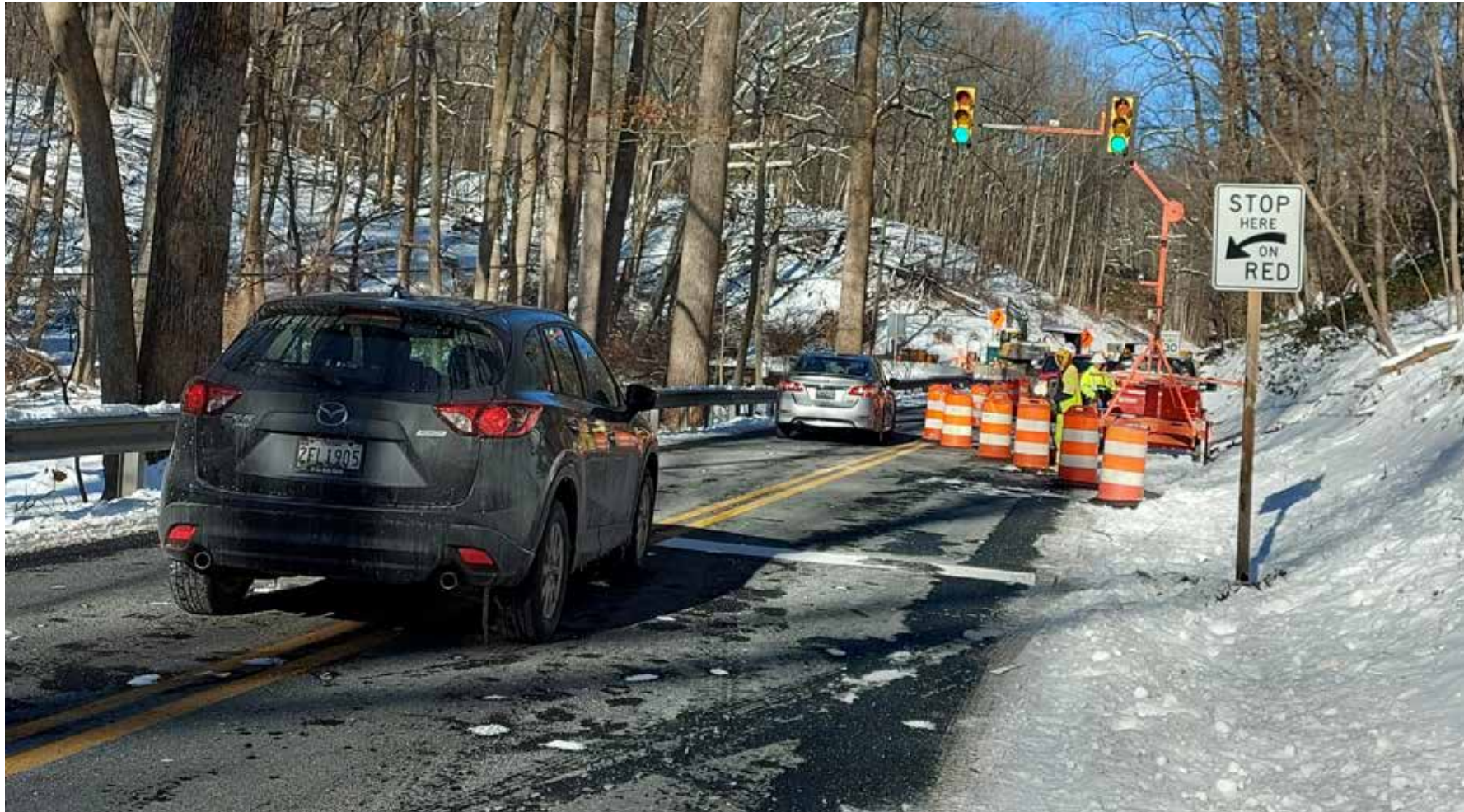
Temporary Traffic Signals for Maintenance of Traffic
