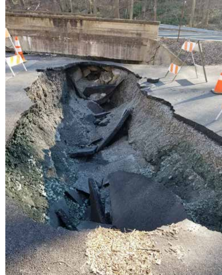
January 2021 – Washout and Pavement Failure
