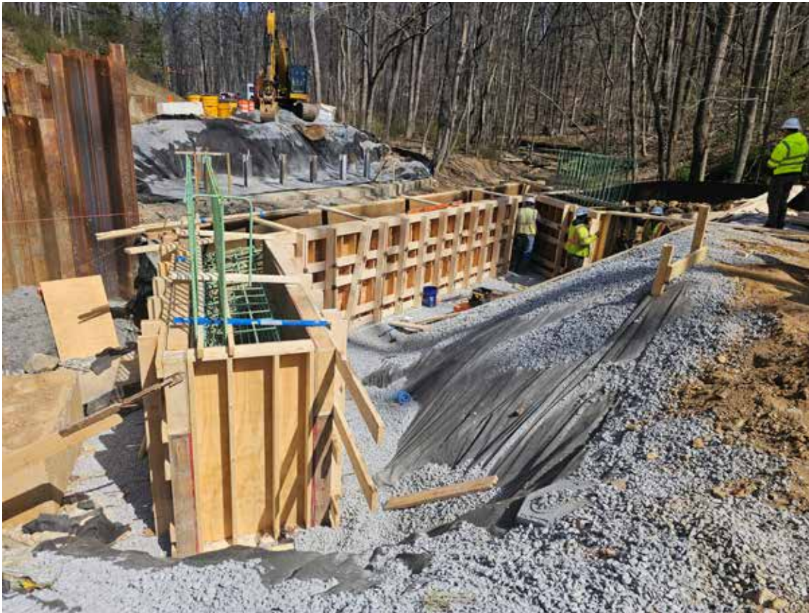
Abutment Formwork
