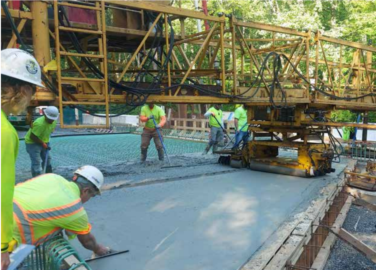
Concrete Overlay Construction
