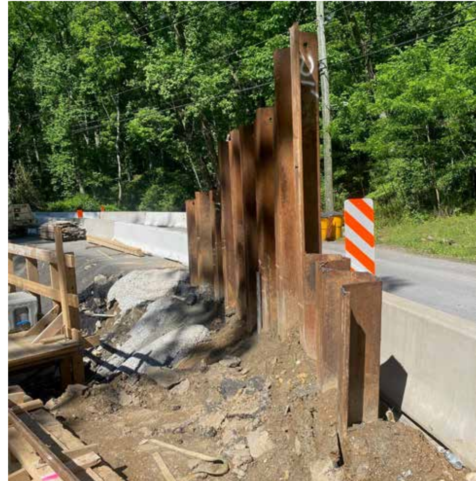
Bypass Road for Maintenance of Traffic / Temporary Support of Excavation
