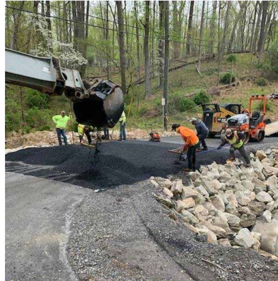
September 2020 – Emergency Repairs
