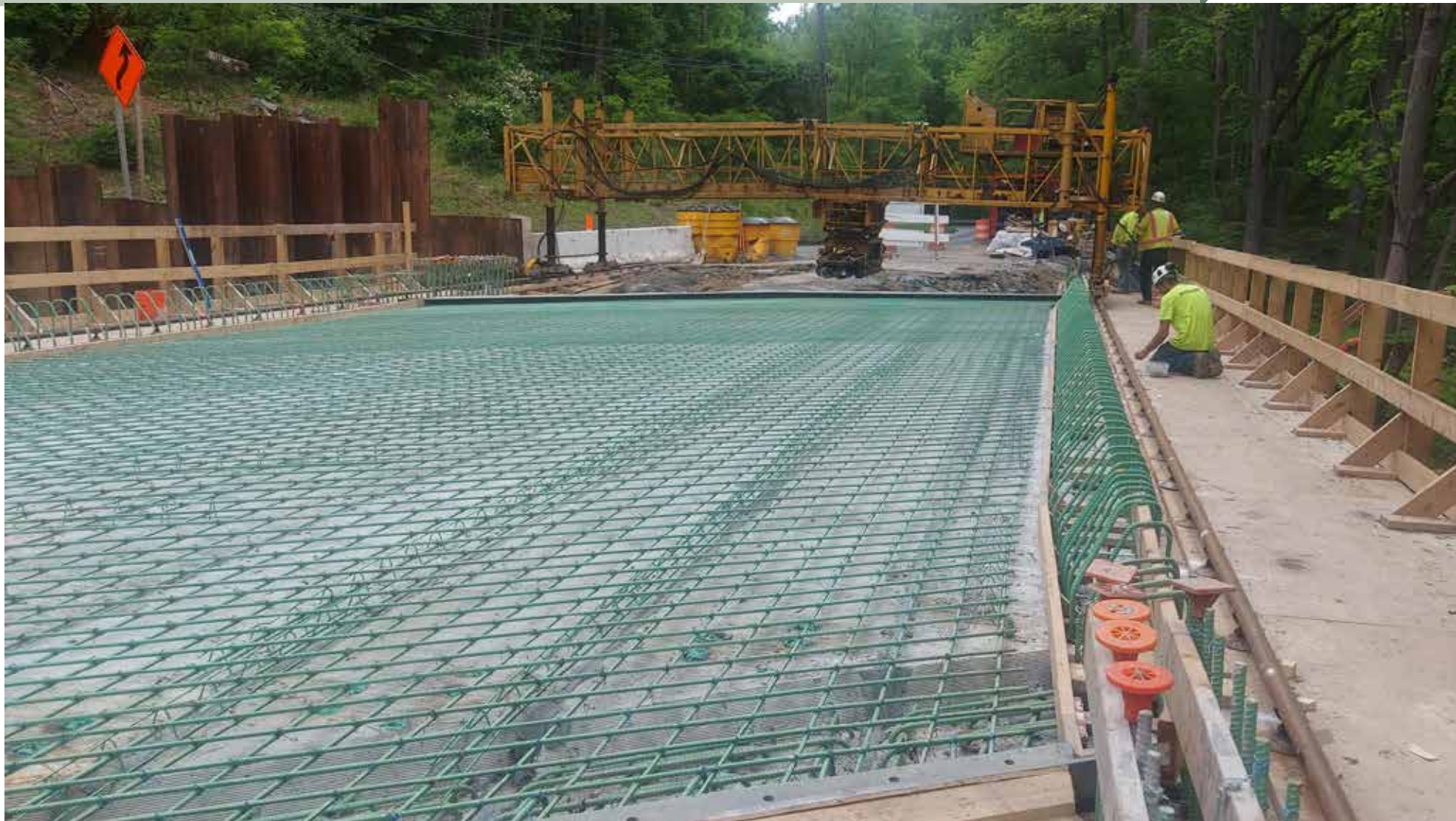
Concrete Overlay Construction
