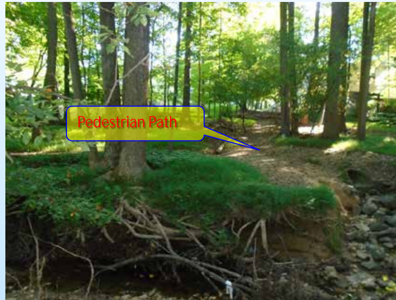
Original “At-Grade” Stream Crossing (looking east towards Auth Lane)
