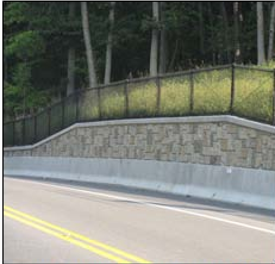
Retaining Wall to Avoid Septic System
