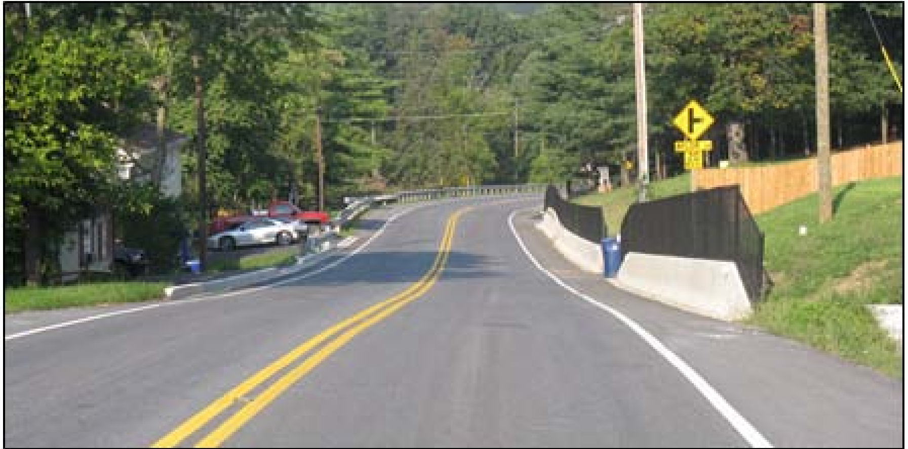
Narrow Shoulder and Curb to avoid Impacts to Homes
